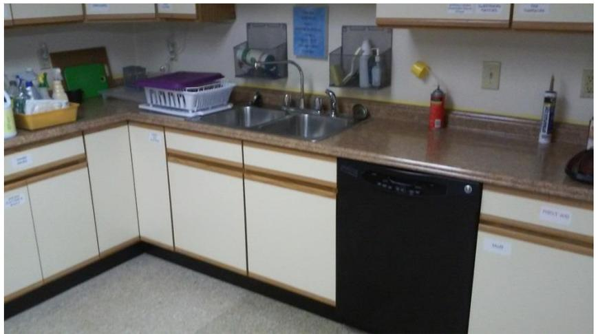
Not related to the hurricane but coincident with drying out the carpet, repairs were made to long-term water damage from a leaking sump pump in the kitchen where particle board had turned to mush or warped. The bases and bottom shelves of some cabinet sections and the counter tops for the whole kitchen were replaced.
